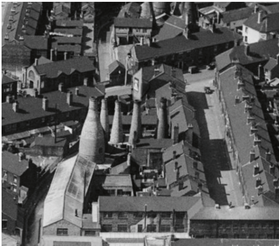
Fig. 20. View of the Warrington Pottery in 1952, looking north-east showing a lightweight structure or lean-to around the southernmost of the ovens. Britain from Above: EAW 045911 © Historic England.
