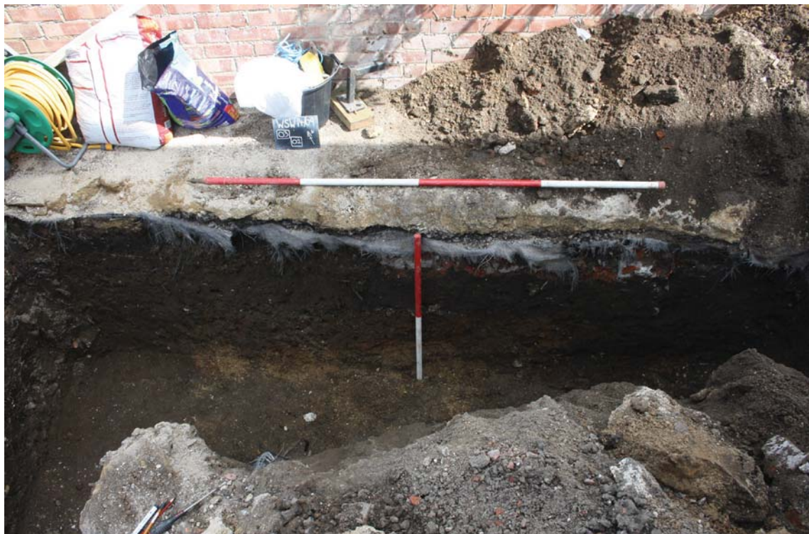
Plate 2. South facing section, showing cut 2 and 3, looking north, Scales: 2m and 1m.
