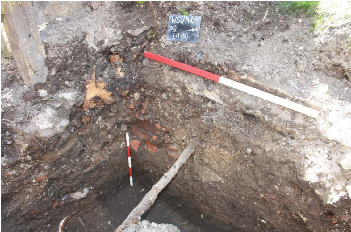
Plate 1. Corner of new footing, darker fill (51) under overburden (50), looking south west, Scales: 1m and 0.5m.
