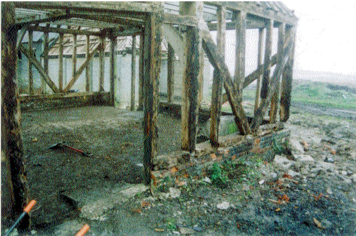
Plate 4. Horizontal timber resting on brick plinth
