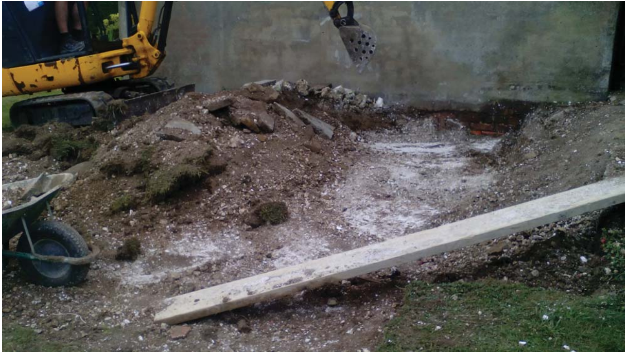
Plate 1: General view of site stripping, looking west
