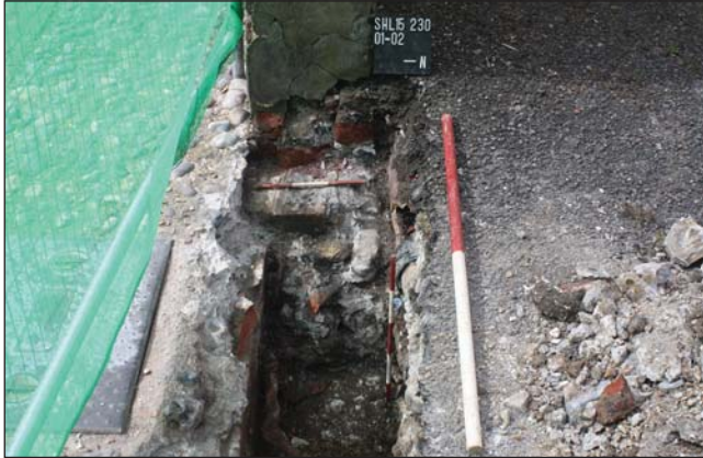
Plate 1. Existing wall 1 and buried wall 2, looking West. Scales: 1m, 0.50m and 0.30m
