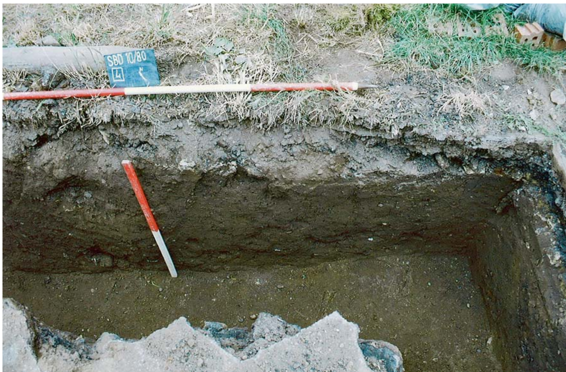
Plate 2. Eastern end of northern footing, looking north-east; horizontal scale 2m (1.5m shown) vertical 1m
