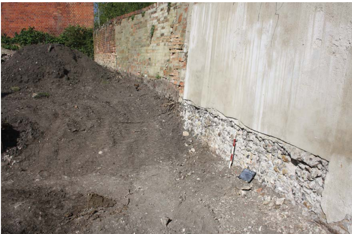
Plate 2. Exposed coursing on northern boundary wall, looking north west, Scale: 0.5m.
