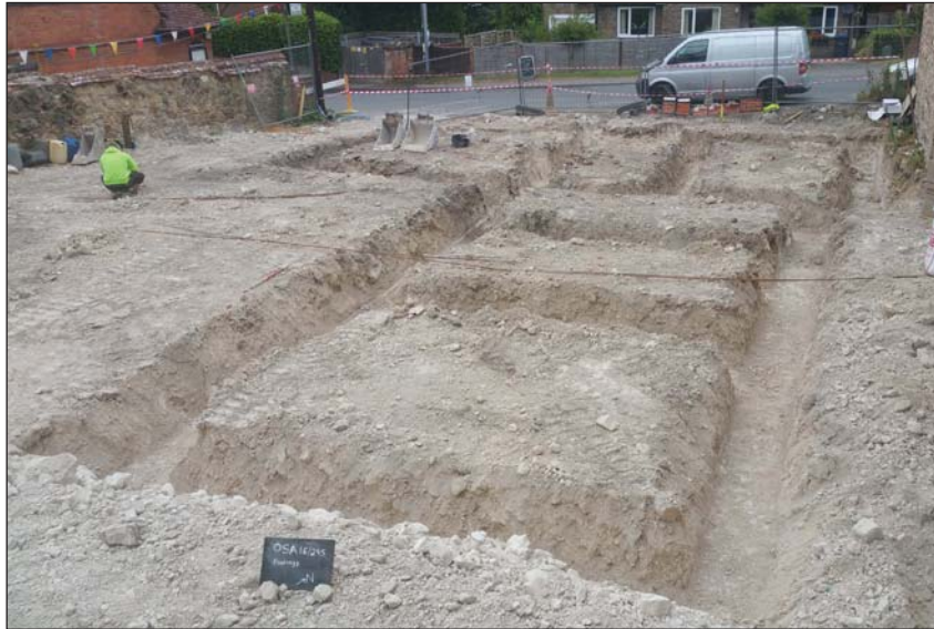
Plate 3. The excavated footings, looking north west.
