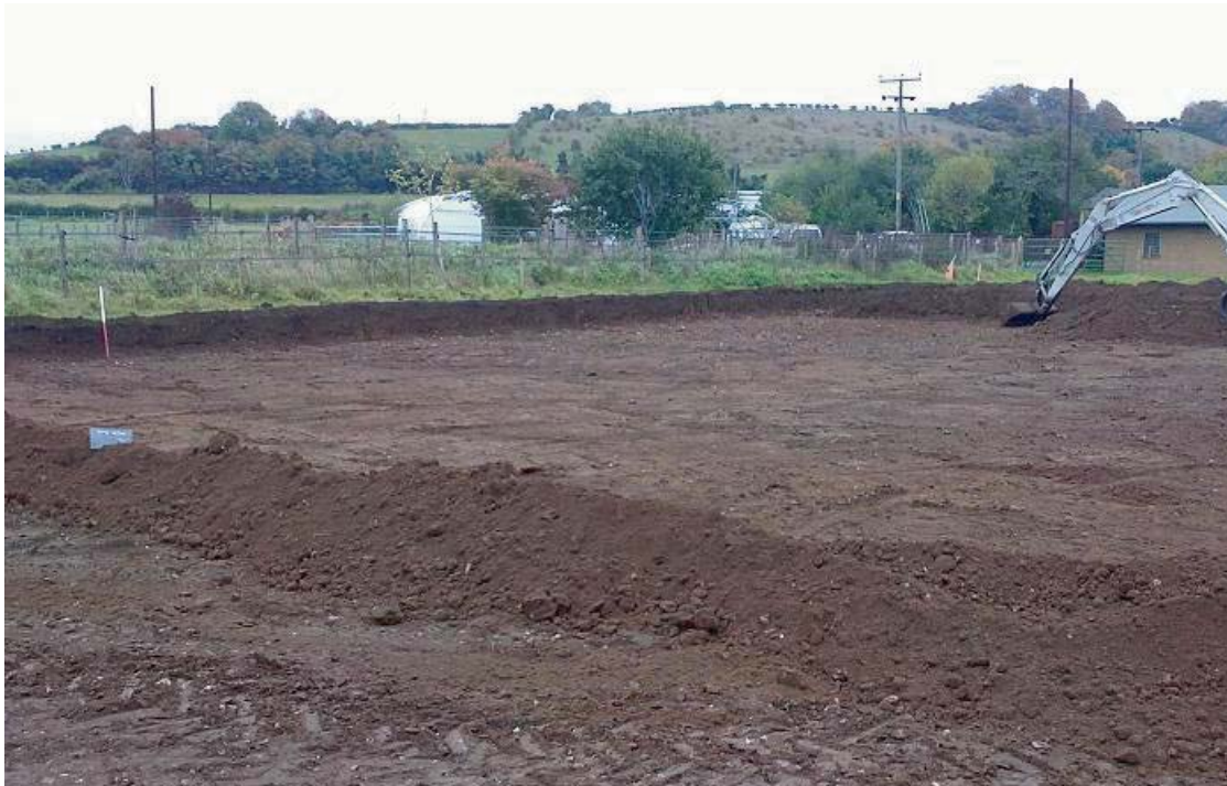
Plate 2. Final level of strip looking north east, scale, 1m.
