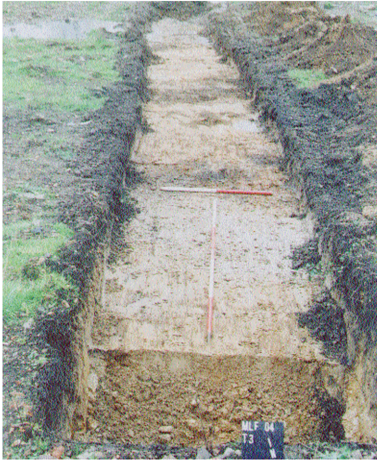
Plate 1. Trench 3. Looking south, scales 2m and 1m
