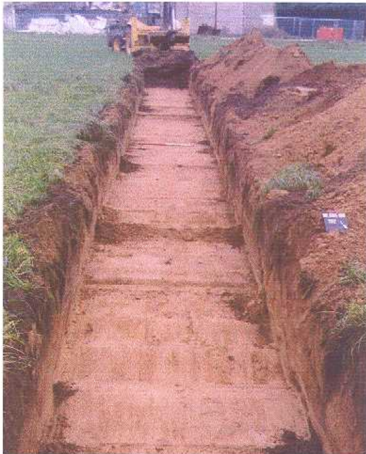
Plate 2. Trench 3, Looking south west. Scale: 1m
