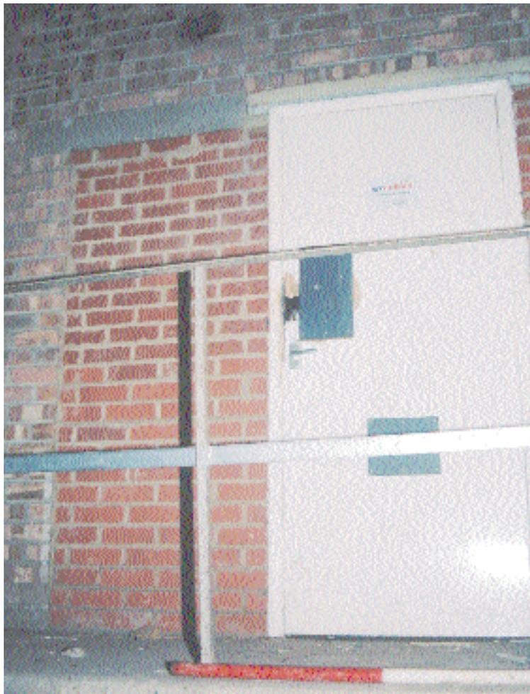
Plate 3. First floor landing with blocked original opening, scale 1m.
