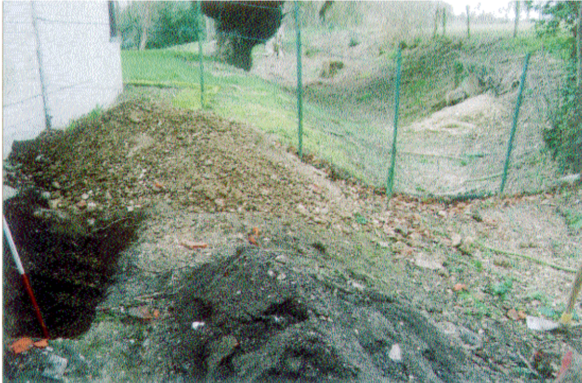
Plate 3. Trench 1 and setting of site looking north east.
