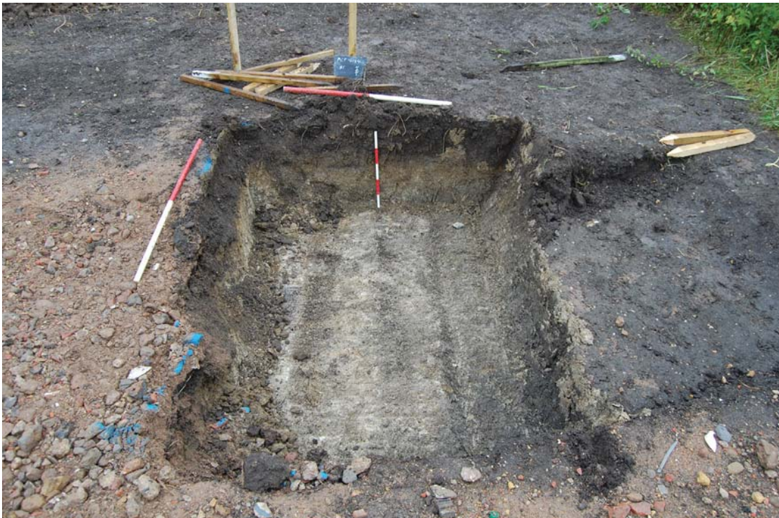
Plate 1. Footing pad 1, looking north, Scales: 1m and 0.5m.
