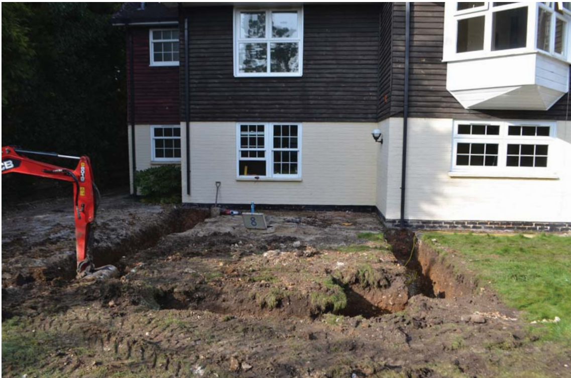
Plate 1. Western footing under excavation, looking north.
