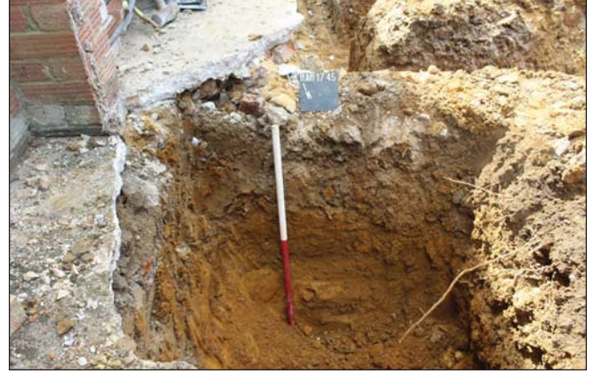
Plate 2. North-eastern footing trench, looking South. Scale: 1m.
