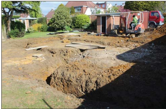
Plate 3. General view of site, looking North-west.
