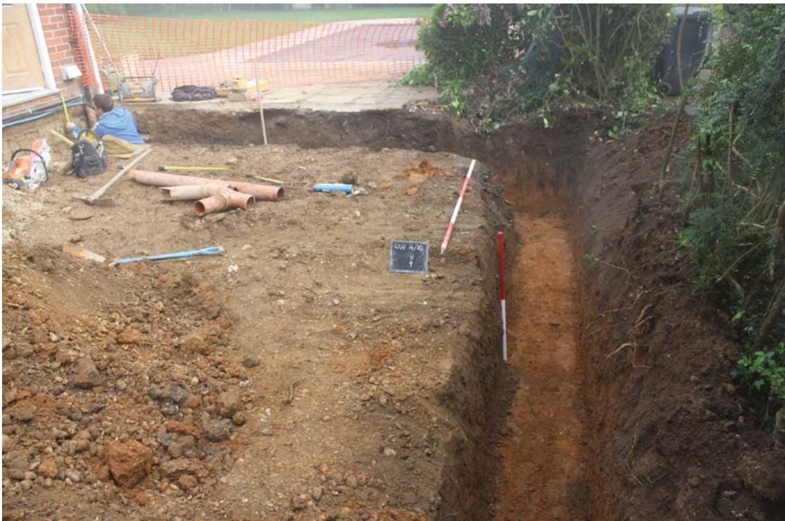
Plate 2. Eastern extension trenching, looking north, Scales: horizontal 2m, vertical 1m.
