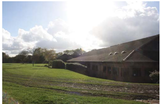
Plate 2. Terracing of school into interior of earthwork.
