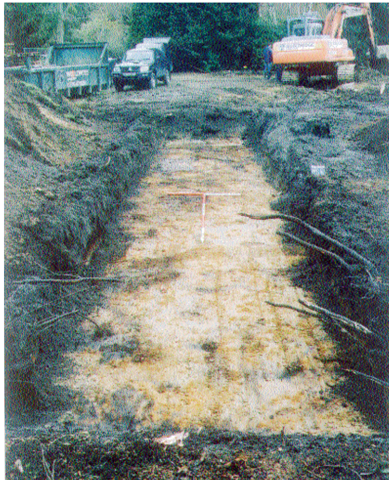
Plate 2. Trench 2 looking north, scales 2m, 1m.
