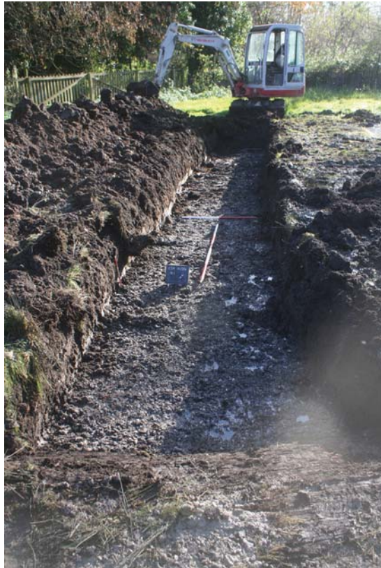
Plate 1. Trench 1, looking north west, Scales: horizontal 2m and 1m, vertical 0.3m.
