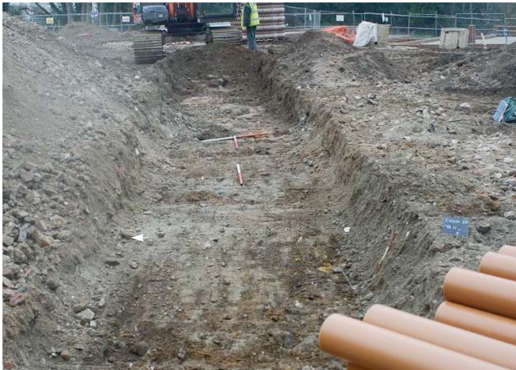
Plate 4. Trench 11, looking north; Scales: 1m and 0.3m
