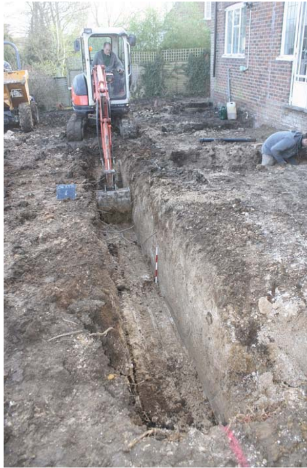
Plate 1. Footing trench under excavation, looking south, Scale: 0.5m.
