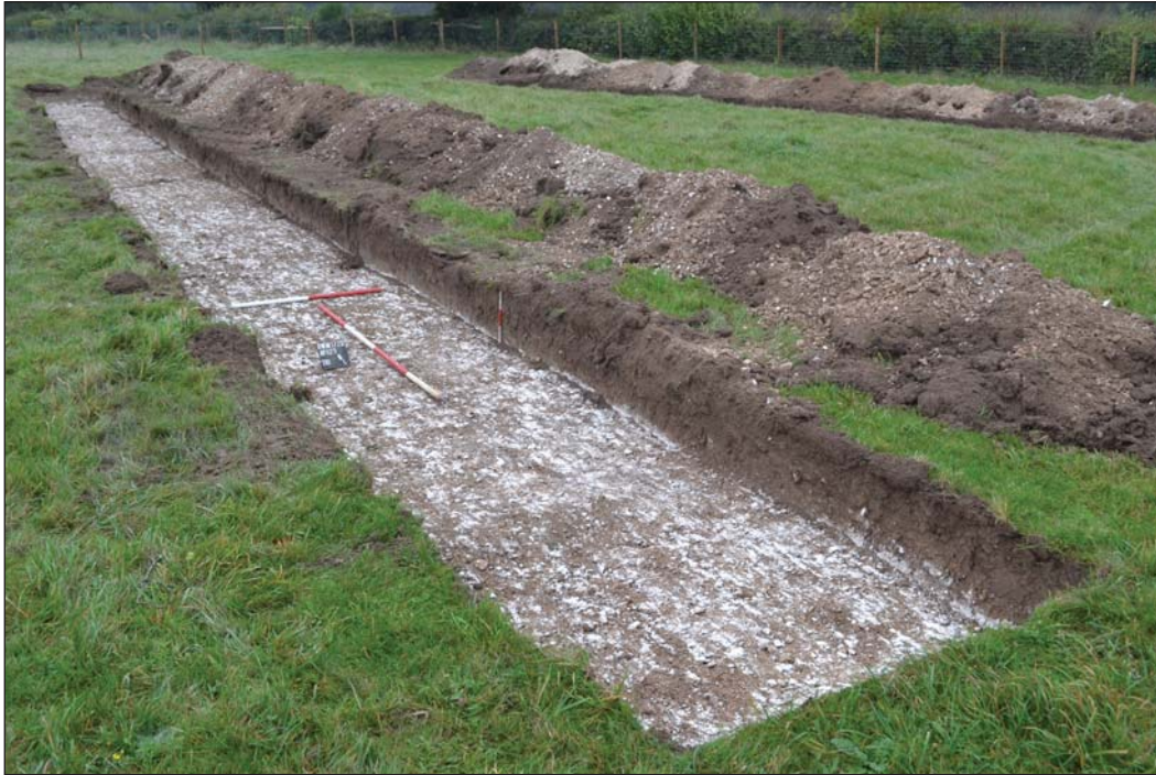
Plate 1. Trench 1, looking north east, Scales: horizontal 2m and 1m, vertical 0.3m.
