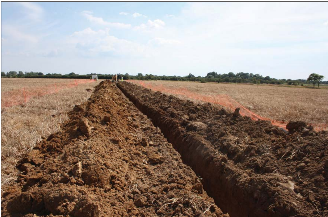
Plate 2. Cable Trench 1, looking north.
