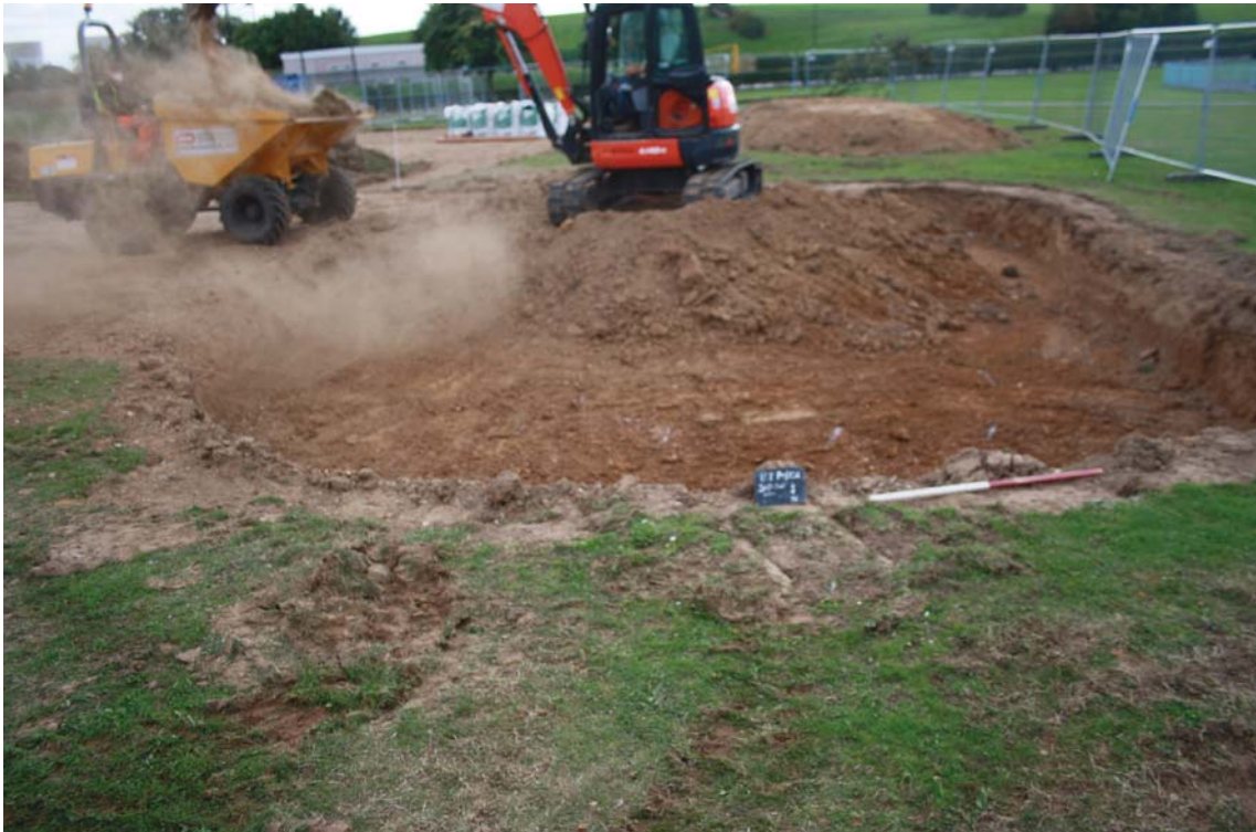
Plate 1. Skate bowl excavation, looking south, Scale: 1m.
