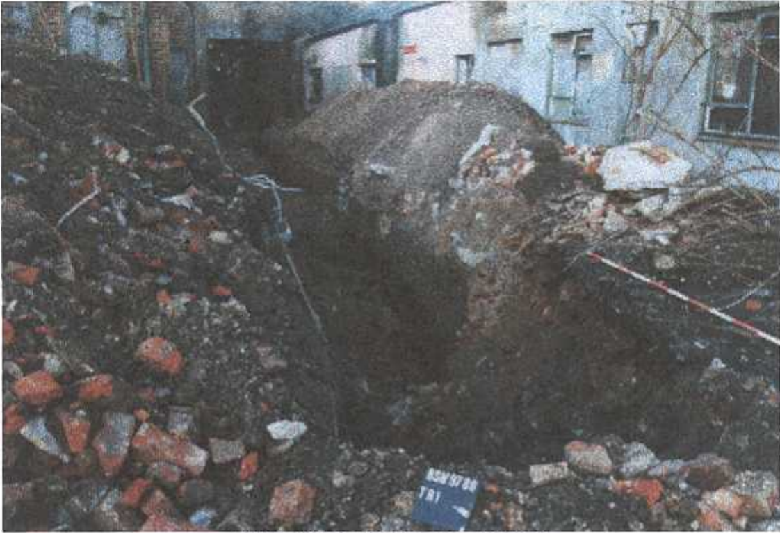
Plate 1. Trench 1 looking west, scale 2m.
