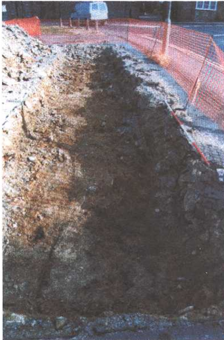
Plate 3. Trench 4, looking north, scale: 2m
