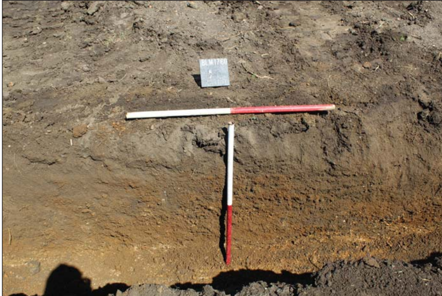
Plate 4. Section of footing, looking north, Scales: horizontal 1m, vertical 1m.
