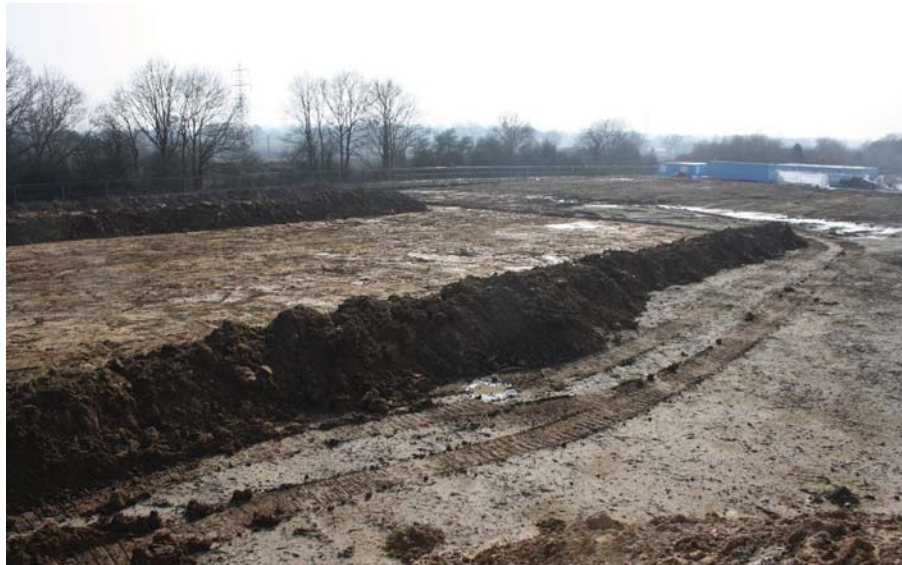
Plate 1. Stripped area, looking south west.
