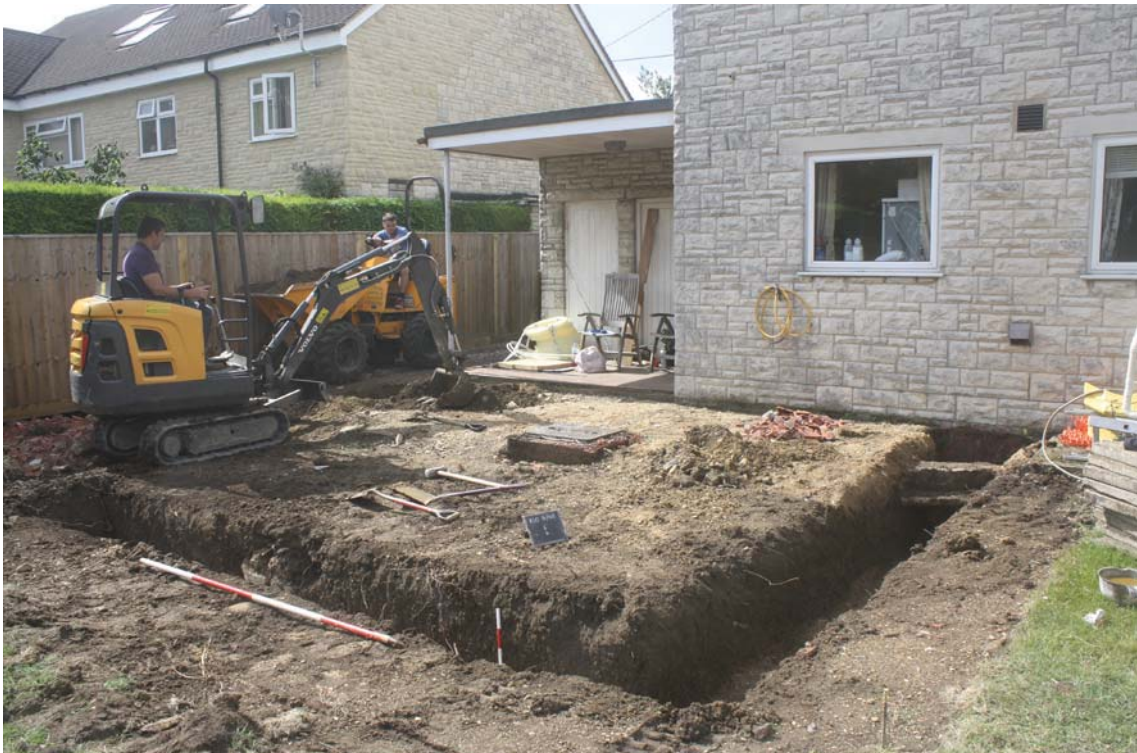
Plate 1. New footings, looking south, Scales:2m.
