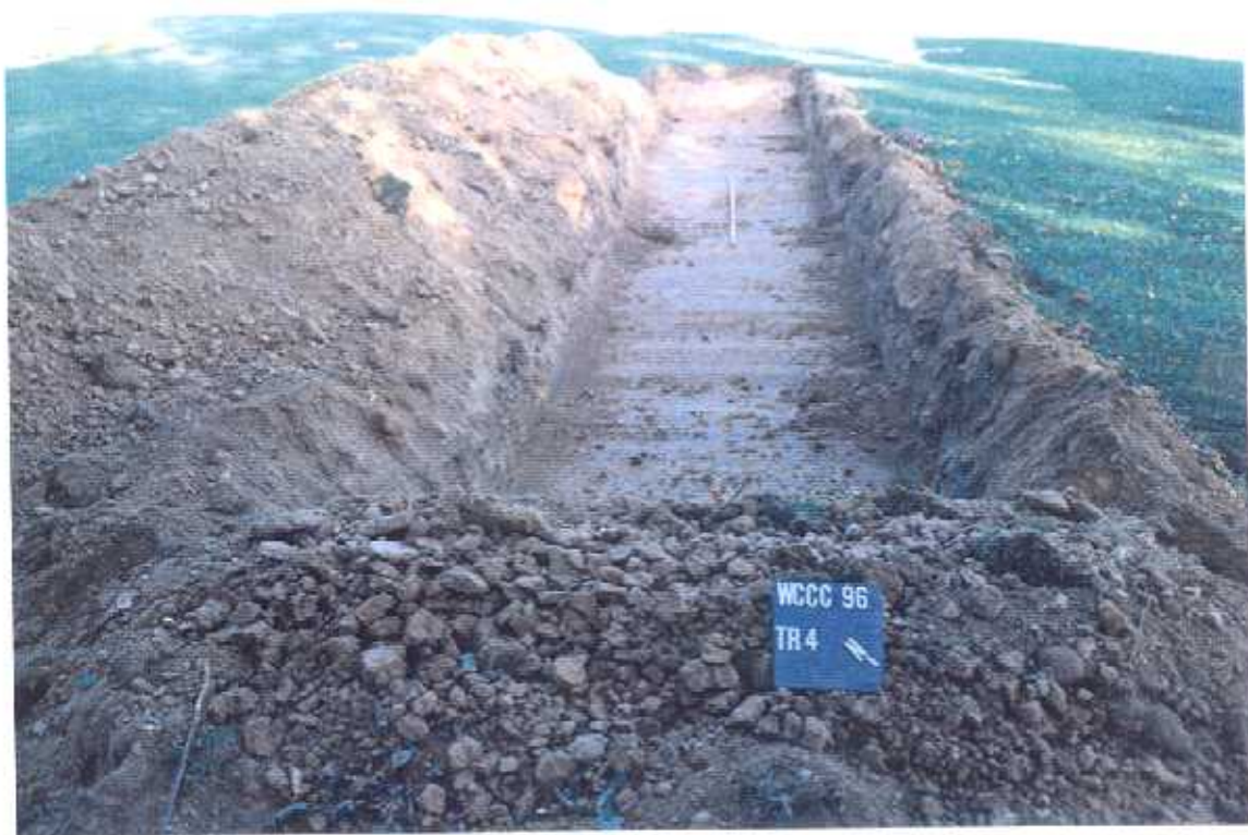
Plate 2. Westergate Community College Chichester. Trench 4. Looking north east Scale 2 m.
