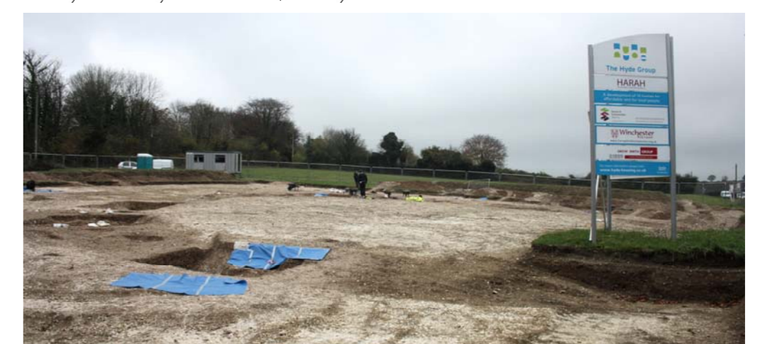
Right: The ring ditch during excavation.
